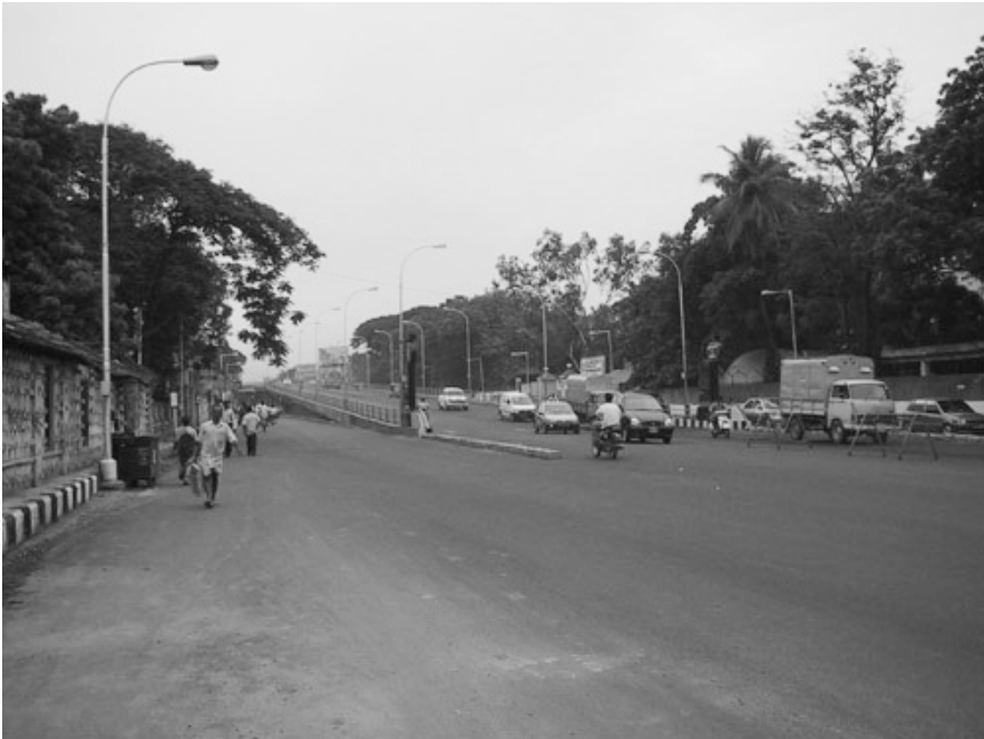
Fig. 2-19 The sidewalk was removed due to the widening of the road (taken in 2000).
