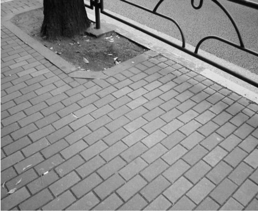
Fig. 2-26 The surface of the sidewalk was changed from paving stones to asphalt at the time of the All-Campus Joint Struggle movement in the 1960s and early 1970s. Recently asphalt has been again replaced by flagstones, but they are strongly fixed. This replacement may be regarded as an act of double hiding by which the historical memory of having repressed the street struggles after the 1960s would be deleted.
