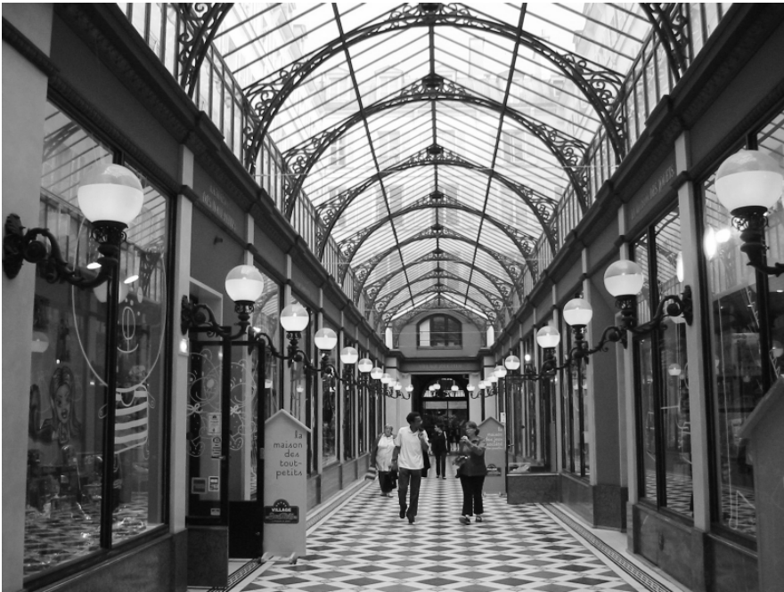
Fig. 2-27 The Passage des Princes in Paris: it has been beautifully renovated and it has become a mall entirely dedicated to toys, the “village of toys.”
